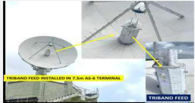
Triband Feed installed in 7.5m Antenna
