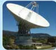
Earth Station Antenna & Electronics
